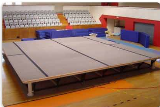
STAGE 3 MATS INSTALLATION
